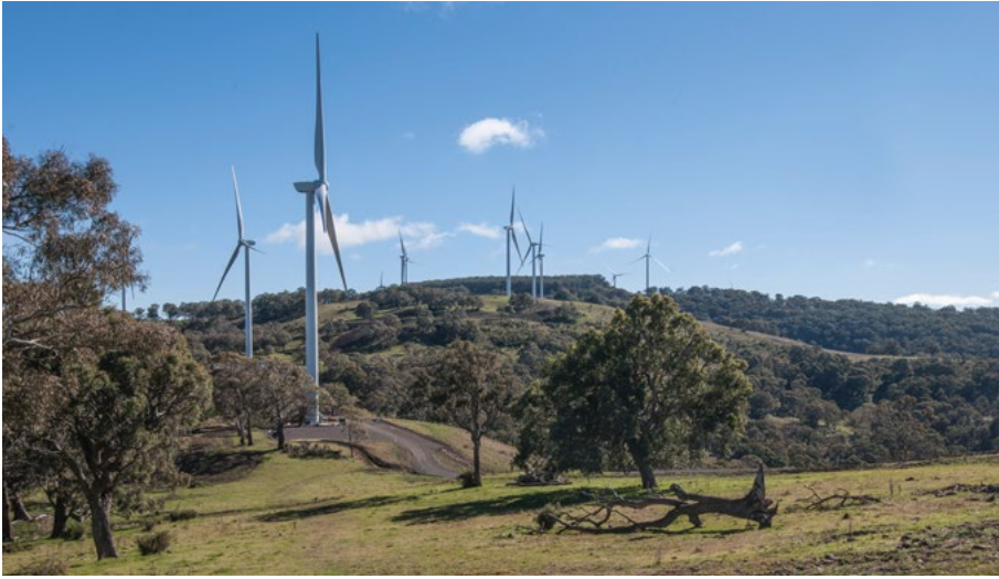
WHITE ROCK WINDFARM
